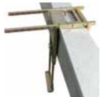
8. Attach compatible tie-back rope to Suspension Bar on The Rack. Then, attach tie-back rope to certified anchor point with minimum breaking strength 5,000 lbs. **THIS ANCHOR POINT MUST BE DIFFERENT THAN THE ANCHOR POINT THE SAFETY LINE IS ATTACHED TO.**
