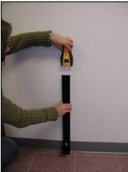
**1-** Using a stud finder attach bottom section of True Plumb to a stud. If base molding is over 1/4" thick the bottom part of the True Plumb must be mounted above base molding. Note: When mounting to a concrete wall use a 1/4" masonry bit and expanders provided.
