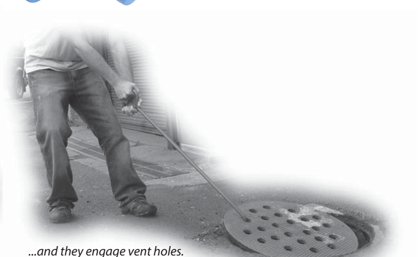
Manhole Hooks engage pick holes...
